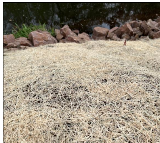
Figure 4: Close-up of Curlex I application.
