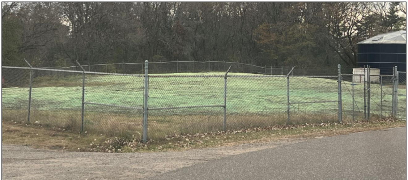
Figure 8: Bindex Wood WT application on the site's flat and shallow-sloped areas.
