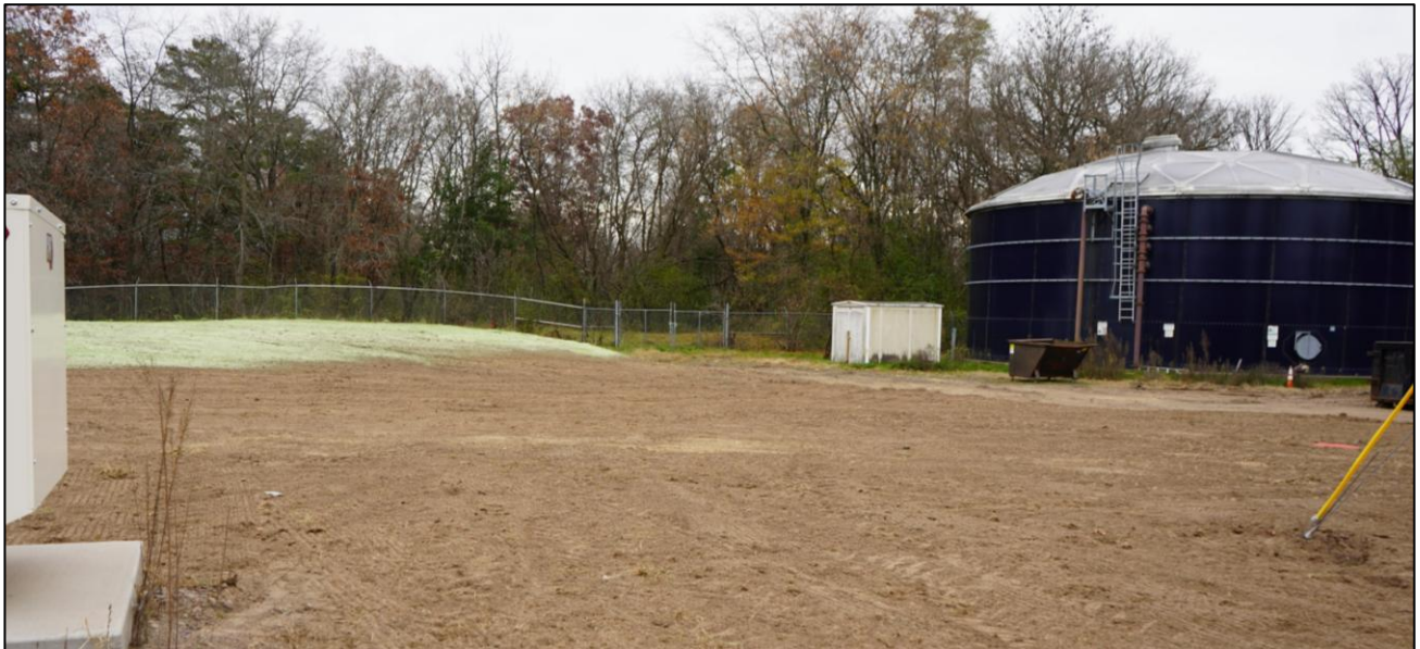
Figure 1: Newly graded bare soil area at the site of the former wastewater treatment plant after the first round of erosion control BMPs was applied.
