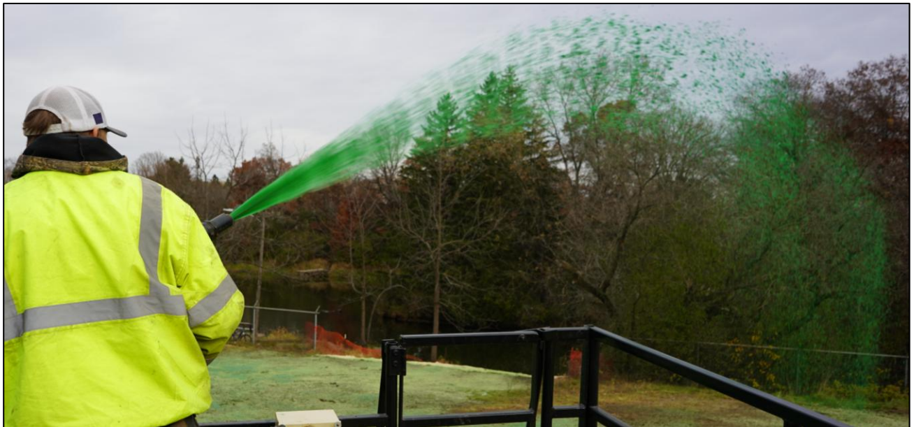
Figure 5: Project personnel hydraulically applying Bindex Wood WT at the site.
