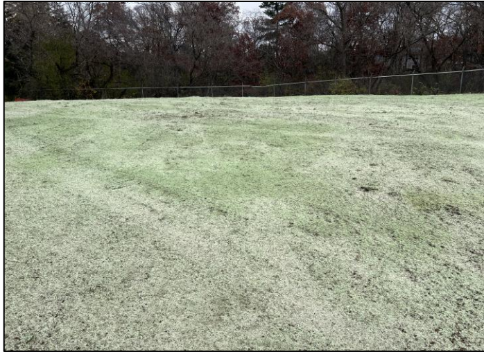
Figure 6: Bindex Wood WT applied on a shallow-sloped area at the site.
