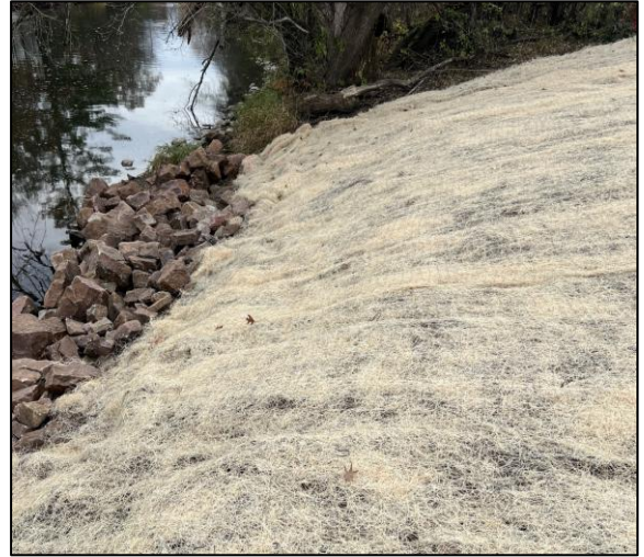
Figure 7: Curlex I installed on the \leq 4H:1V sloped area adjacent to the nearby river.
